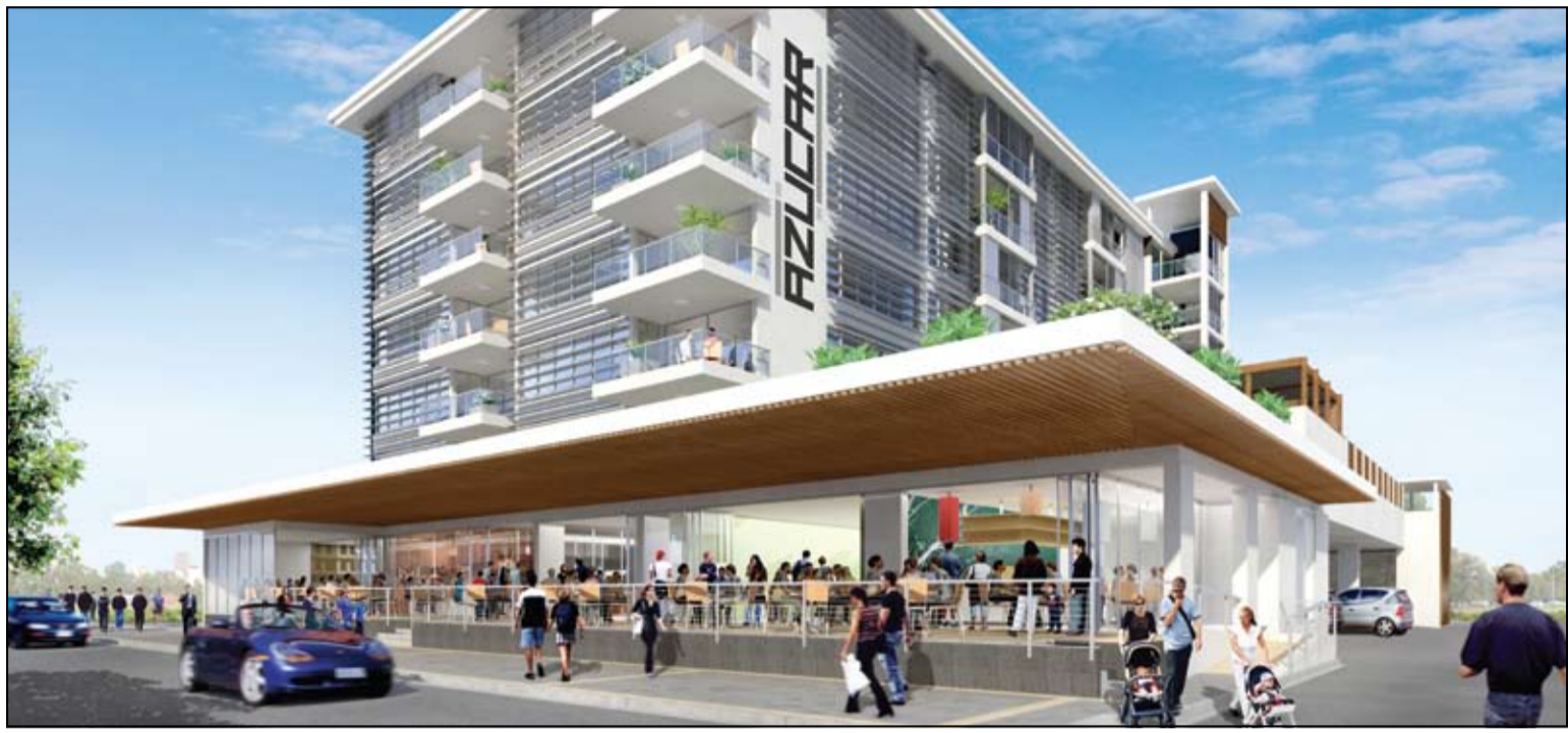
Azucar located in Mackay – a fine example of Honeycombes' prime regional developments.
